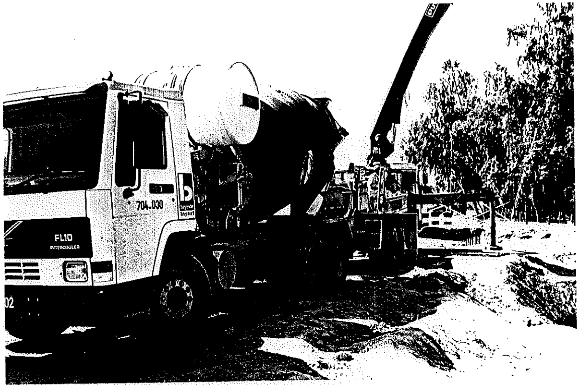
Photo-13 Fresh cement concrete is being poured using pump
