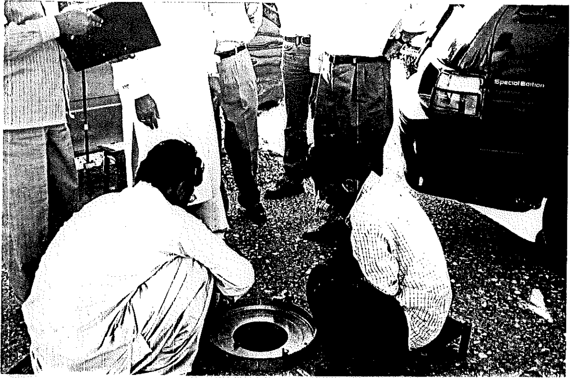
Photo-5 Field density test over base course
