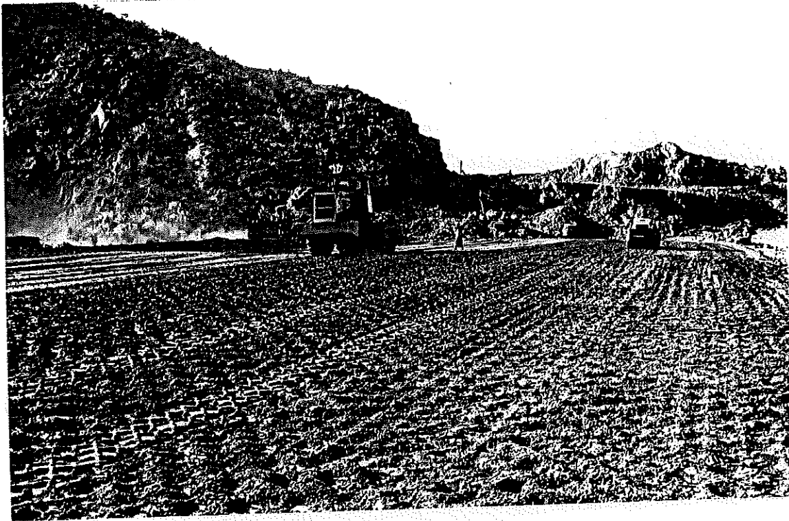
Photo-1 Subgrade preparation underway
