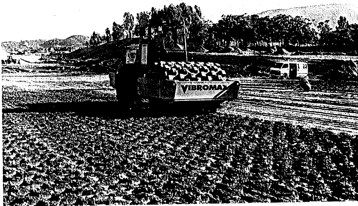
Photo-2 Subgrade compaction using sheep foot roller
